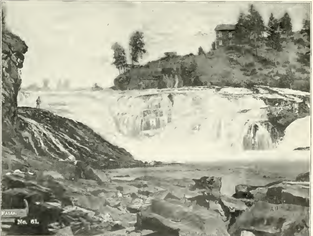
LOWER FALLS OF THE SPOKANE AS THEY APPEARED THIRTY YEARS AGO
